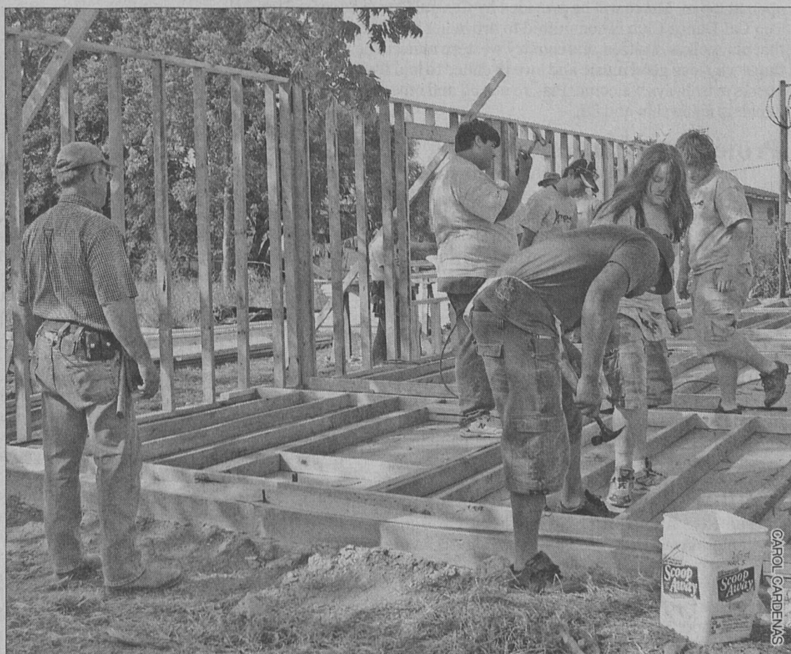
Pictured above are members of St. Paul Lutheran Church of Columbus with prospective homeowner Jessie Upson. Members of the church were there to help start putting up the walls on the home located on State St.
